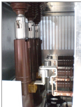
Circuit breaker position: CONNECTED
