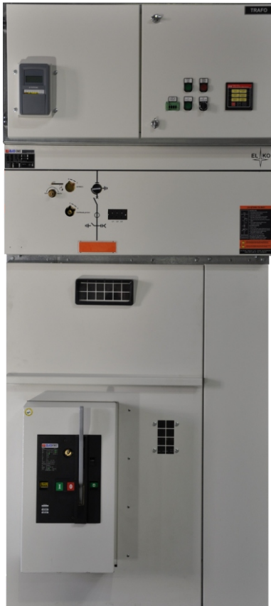
Cubicle with circuit breaker
